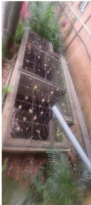
Figure 4-23: RWH sump near dental blocks
