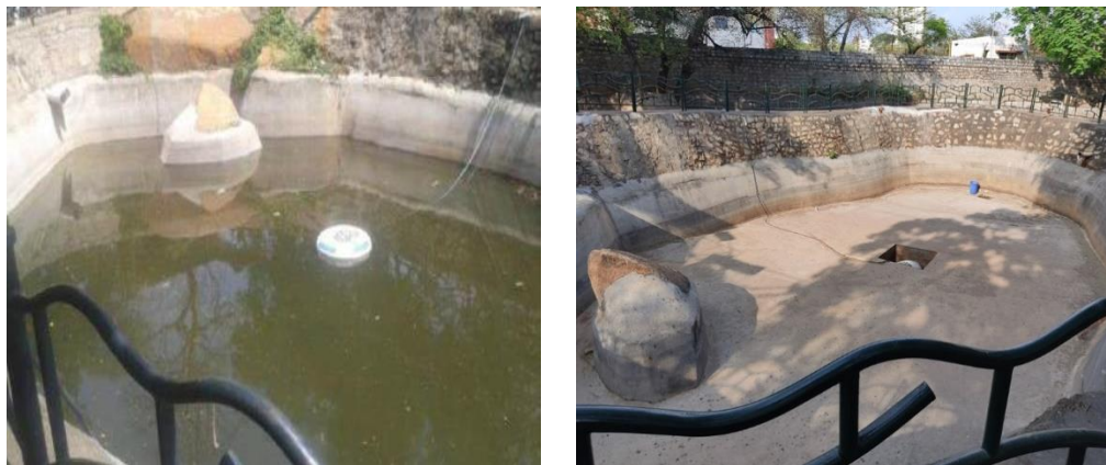
Figure 4-7: Rain water harvesting pond
