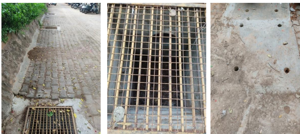
Figure 4-10: Percolation pits for rain water harvesting
